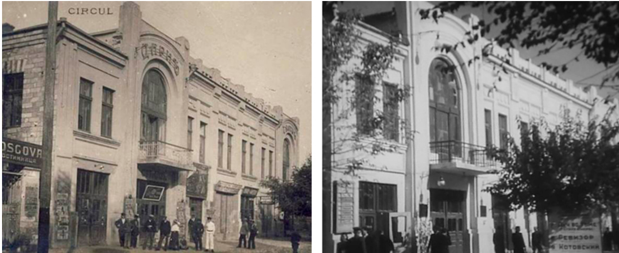
The building that today represents the National Philharmonic was built in 1912 and opened in 1913 as a circus. After more than two decades, in 1940 the institution of the Philharmonic was created, and the headquarters of the former circus became, until now, the home of the National Philharmonic.
