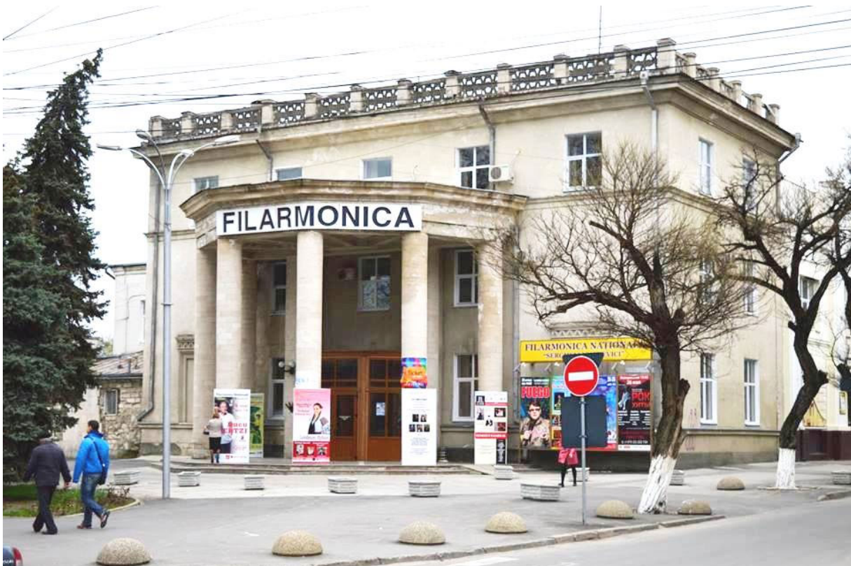
Street view perspective of the building of the National Philharmonic “Serghei Lunchevici” in Chisinau, before the fire on September 24 th 2020.
